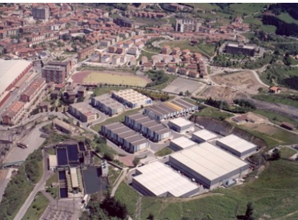
Figure 2 - View of Argixao Industrial Park
