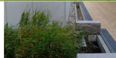
Trincea filtrante - Western Harbour, Malmö
