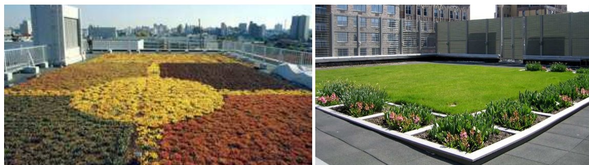
Extensive and intensive green roofs
