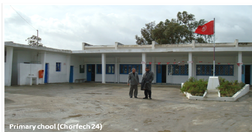
Figure 6 : Primary School of Chorfech
