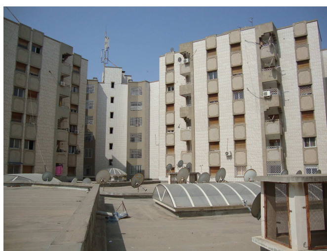
Figure 10 : Part of the Bardo centre building, view from the first floor
