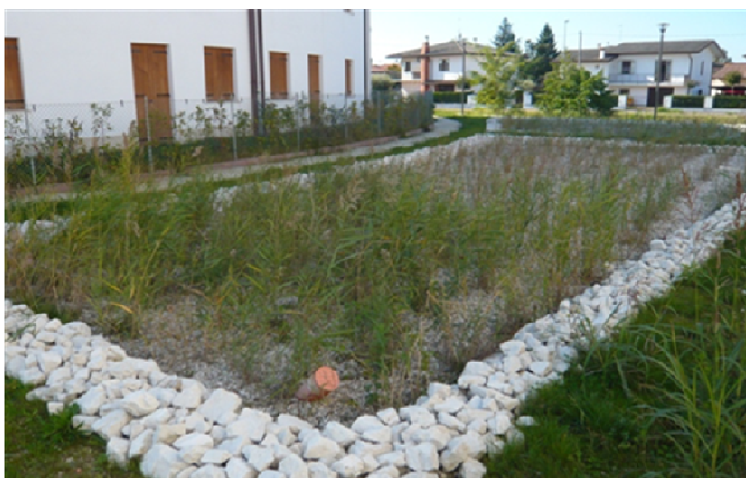
HF system fro greywater reuse in Preganziol (TV) for 240 a.e.
