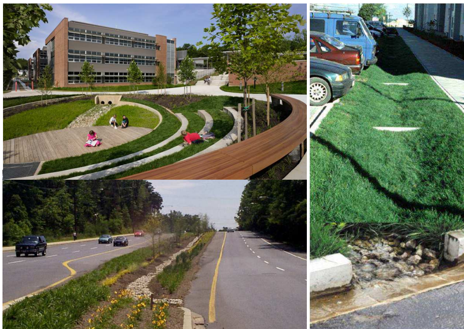
Bioretention area, infiltration trench and vegetated infiltration swales
