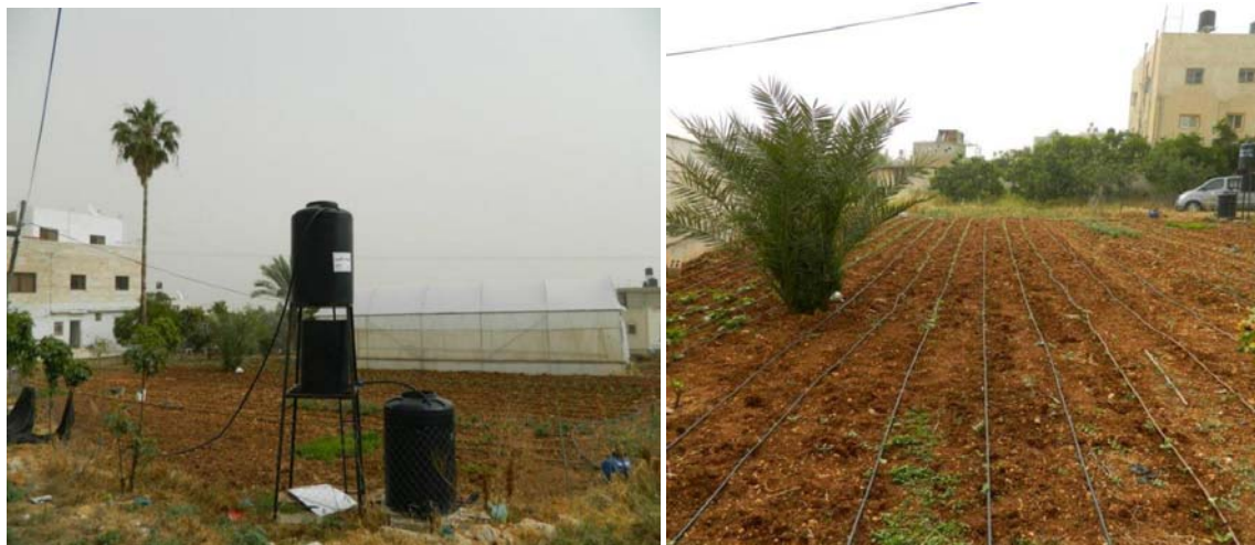
Picture 13 final filtration stage by carbon and gravel filter and reuse for drip irrigation at household level near Ramallah (source: PHG)
