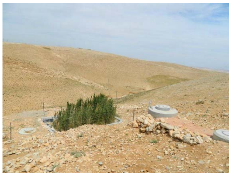
Picture 14 a Vertical flow system for greywater treatment in a Bedouin village of 70 persons near Hebron (source: IRIDRA-Oxfam Italia)
