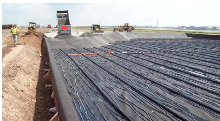
Picture 25 Construction details of the aeration system (source: Scott D. Wallace)
