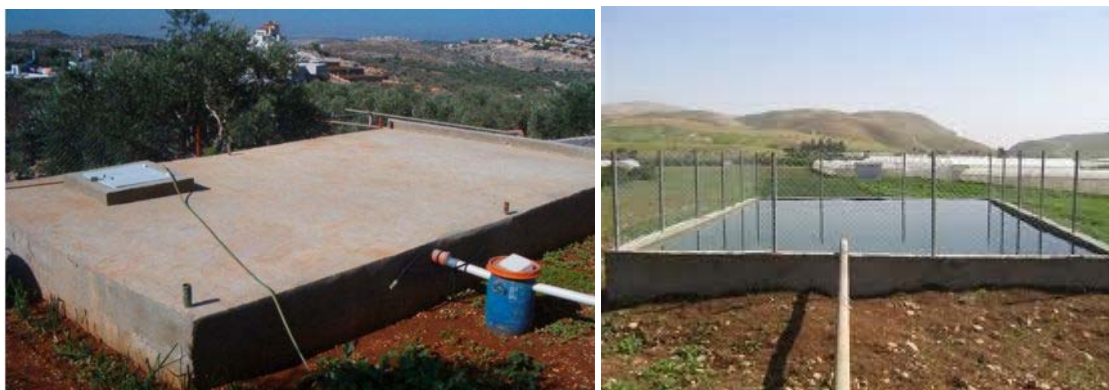
Picture 11 Rainwater harvesting covered and open cisternes in Palestine (source: PHG)
