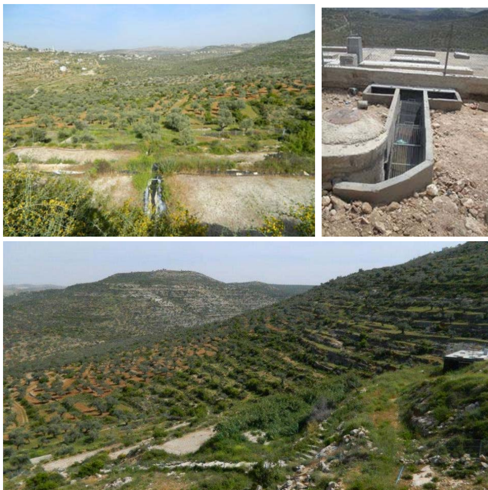
Picture 3 Bani zaid WWTP: screen and UASB (on the left), Horizontal CW (on the right)
