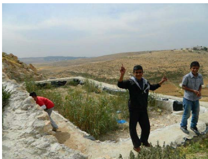
Picture 16 – HF system for greywater reuse in Palestine
