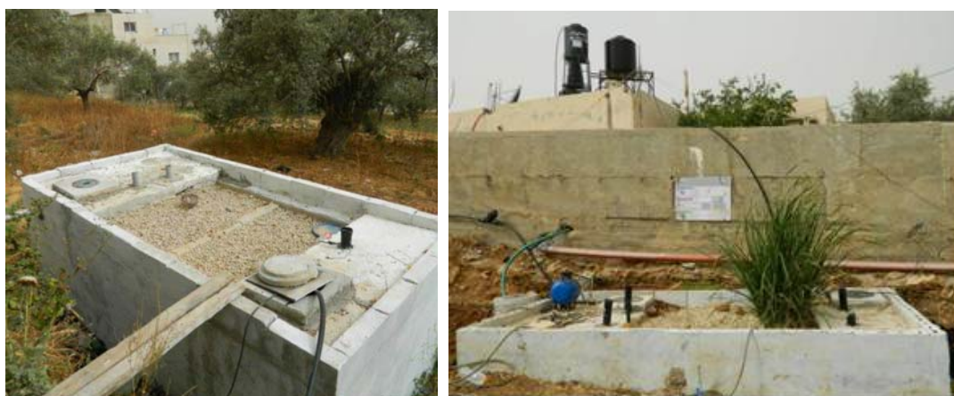
Picture 12 unplanted and planted upflow gravel filter at household level near Ramallah (source: PHG)
