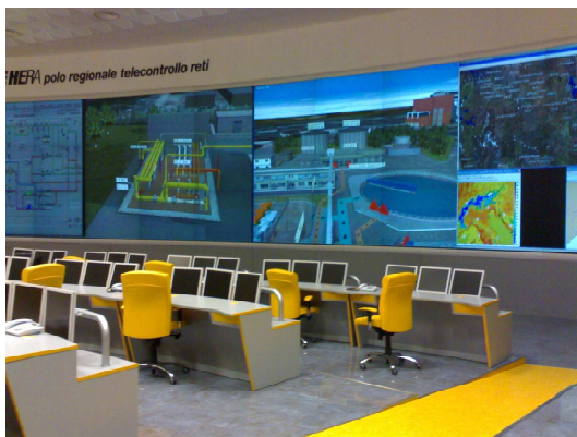
Figure 1 Supervisory Control and Data Acquisition systems of HERA S.p.A. (Italy)
