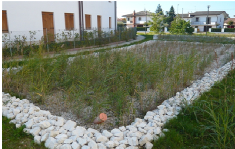
Picture 10 HF system fro greywater reuse in Preganziol (TV) for 240 a.e.
